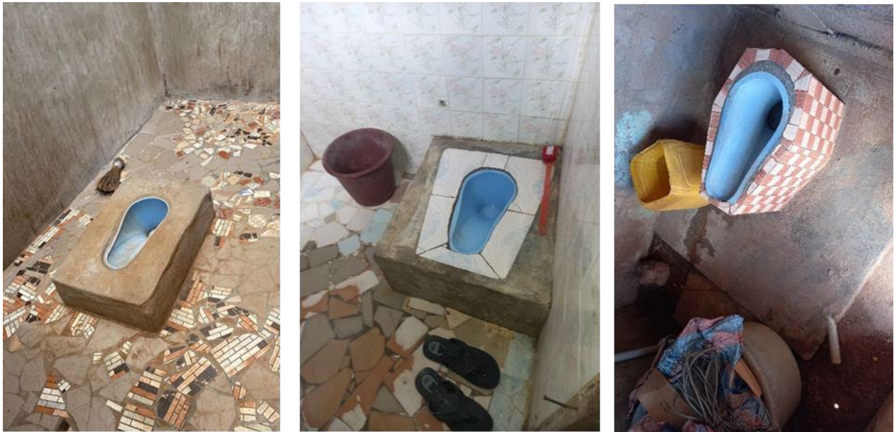
Figure 5: Installation of SATOPan (from left to right: Bouaké, Yopougon, Calavi)
