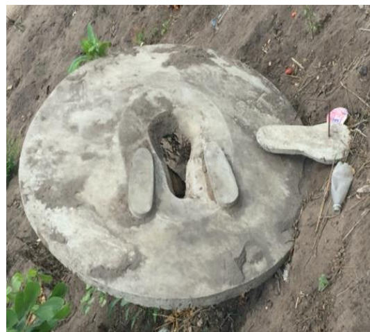
Figure 10: Concrete latrine slab not being used due to technical design issues.
