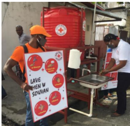
30. Installation of handwashing stations in Archie. Source: HRC
