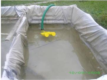
Water pumped from the river into settling ponds made from tarpaulins, treated with alum and allowed to settle.
