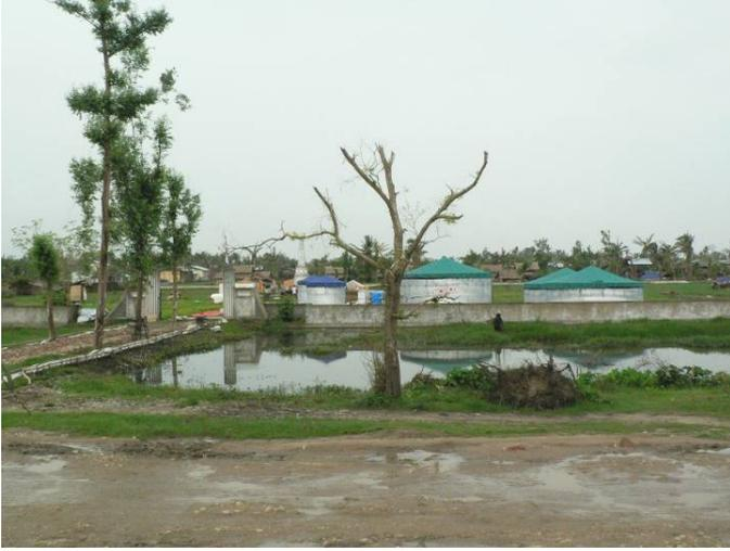
Part of the French Red Cross ERU being used for sedimentation and chlorination.
