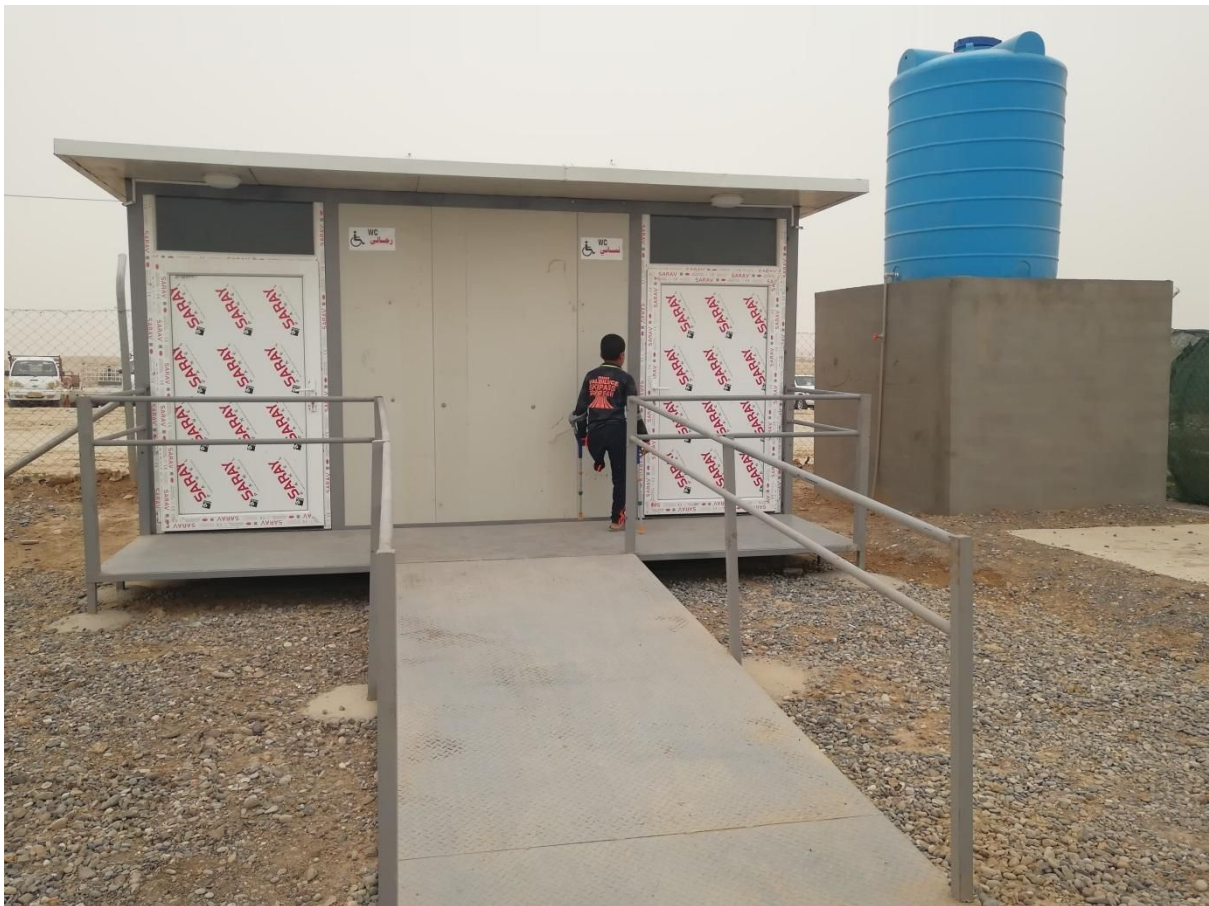
Accessible latrines at the Primary Health Care of Jedaah 6 IDP camp
