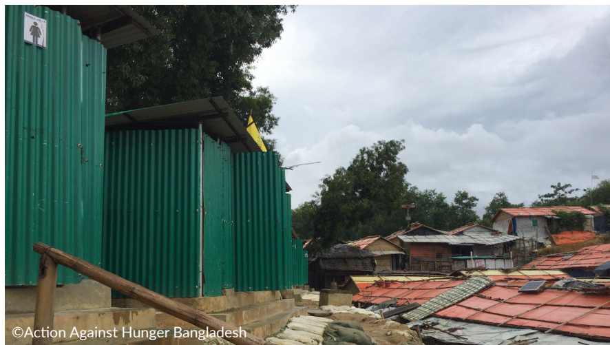
FIGURE 5: ACF BUILT SANITATION FACILITIES IN REFUGEE CAMP
