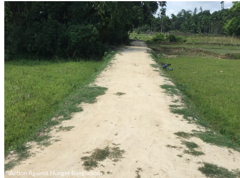
FIGURE 3: A ROAD CONSTRUCTION BY HOST COMMUNITIES CFW RECIPIENTS
