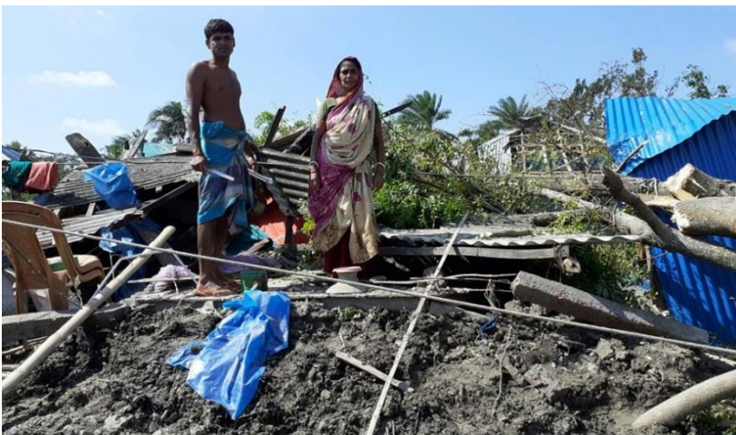
Cyclone bulbul damaged houses at Shyamnagar, Satkhira.
