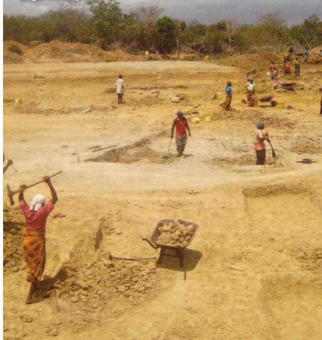
Women and Men in a Kilifi community working on a large water pan
