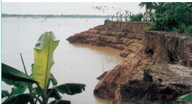
Riverbank erosion is a major concern of villagers in Kampong Cham. The village map clearly shows houses and roads as elements at high risk.
