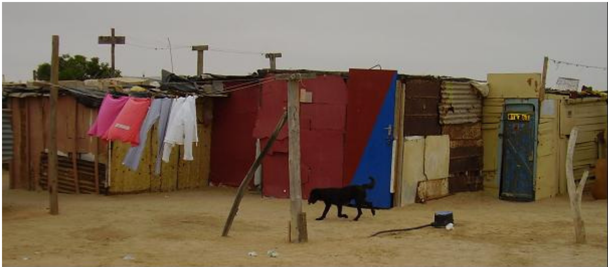
Photo 1 – Informal water supply through metered piping in an African shanty town
