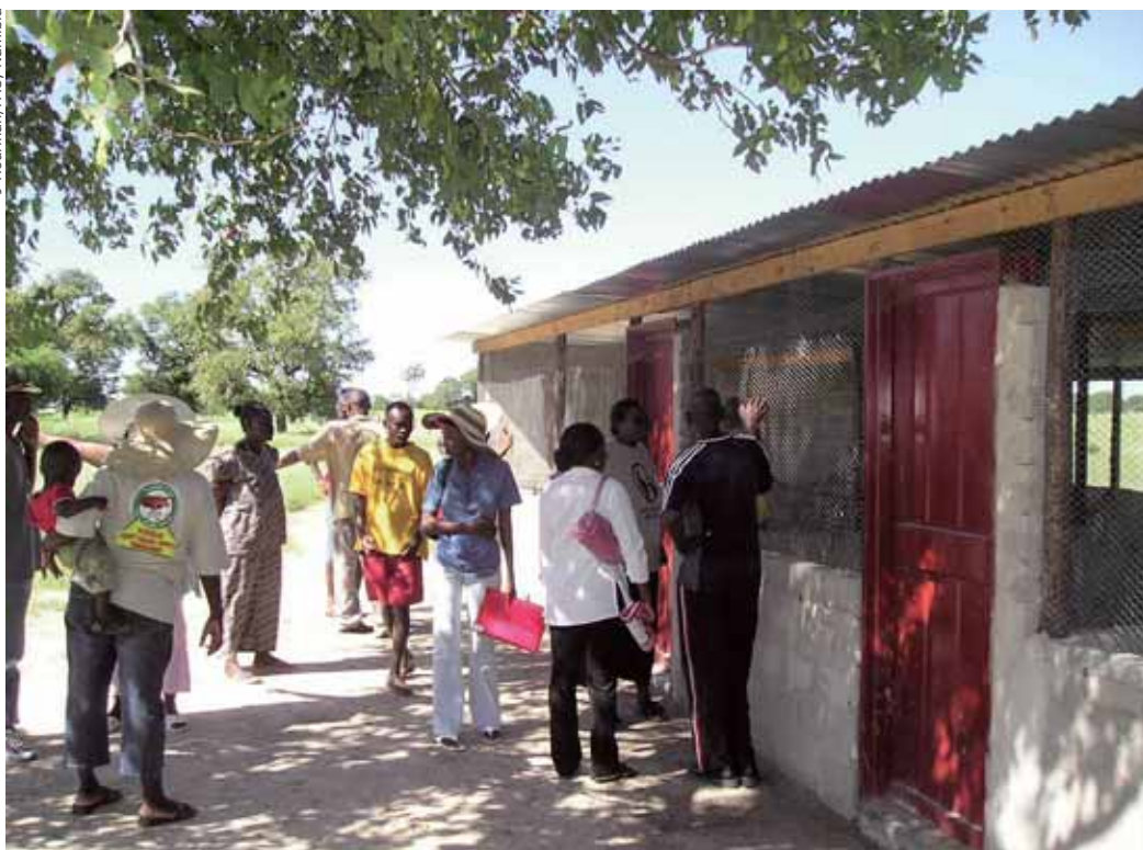
This building houses a chicken and a guinea fowl coop, as well as a space for rabbit rearing, all part of the JFFLS training programme.
