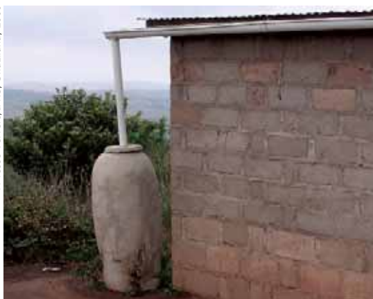
Collecting water from a house roof
