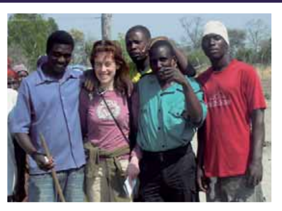
Local youths volunteering to help in site clearing at Seim Nujoma Combined School, Kebbe
