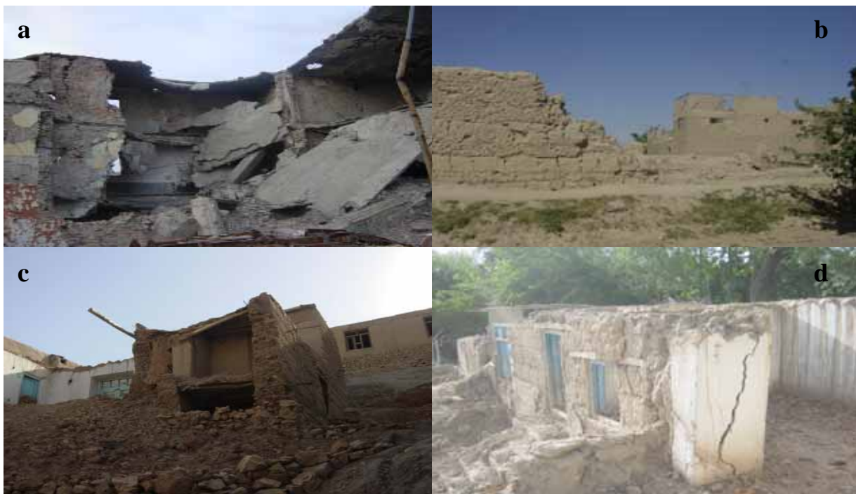
Fig. 4. Photos showing the effect of damages due to conflict in urban areas (a), rural areas (b) and due to natural disaster like earthquake in urban areas (c) and rural areas (d)
