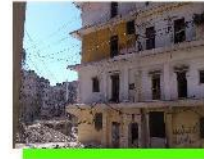
Category 1 (slight damage) Light repairs required (windows, doors)
