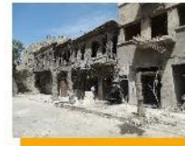
Category 3 (Heavy damage) Over 30% roof damaged Severe fire damage Repair possible
