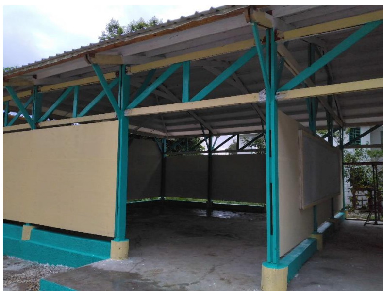
PHOTO N°10: TEMPORARY SCHOOL CONSTRUCTED WITH THE SUPPORT OF UNICEF (LES CAYES)
