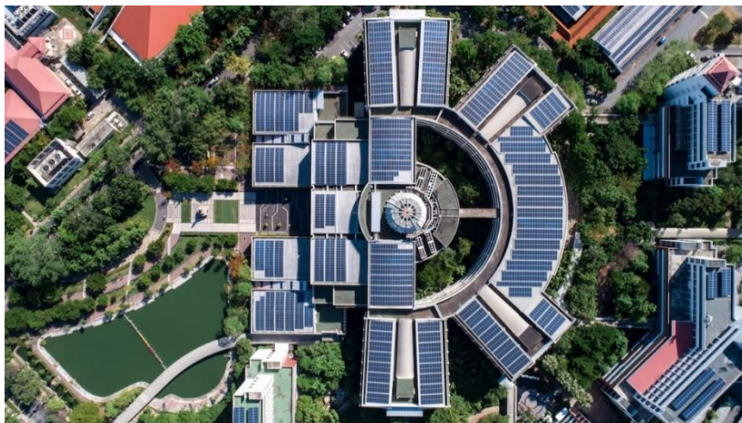
Thammasat University Solar Rooftop, Thailand.
