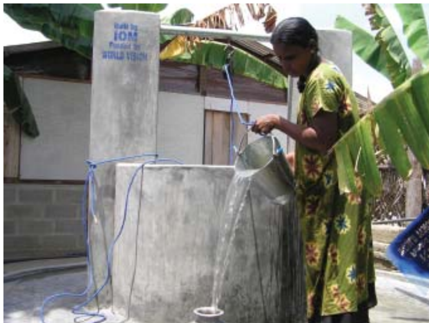
Wells constructed for residents at shelter sites
