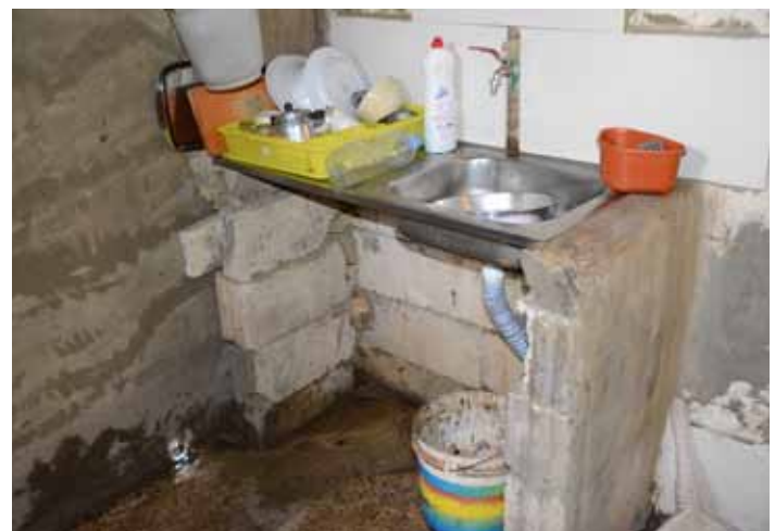
A sink area in a Syrian refugee housing unit in Baabda, Lebanon
