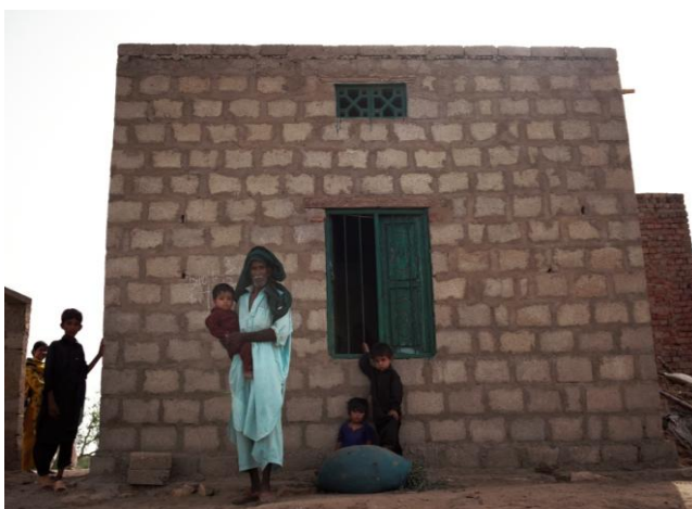
A concrete, more resilient house constructed by ActionAid in Arbab Obhayo village, Sindh
