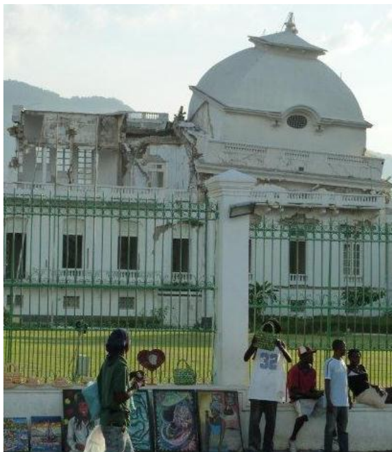
Figure 1 Office of the President after the earthquake
