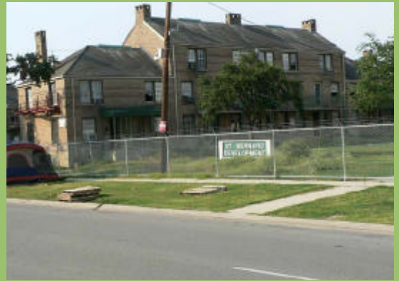
DEMOLISHED : 1,400 units of solid, decent, vibrant, minimally-damaged public housing at the Saint Bernard project.
