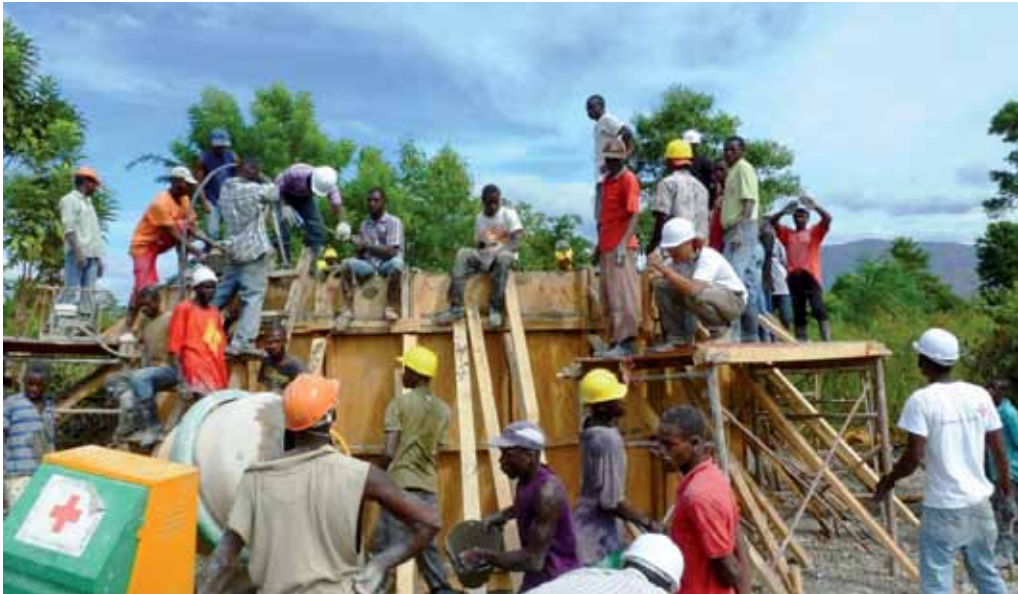
Construction of rural gravity-fed water system in Verrettes, Artibonite.
