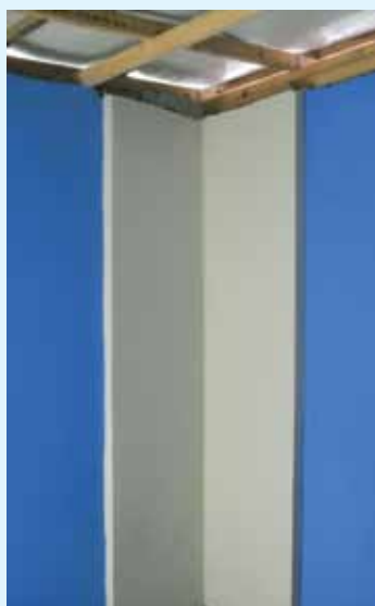
Reinforced corner inside the house
