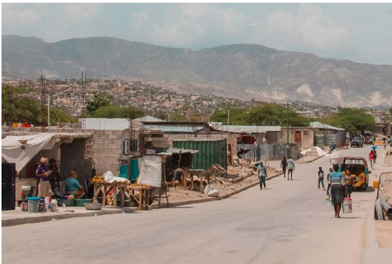
A completed road in Canaan, which utilised UN-Habitat spatial analyses and the participatory urban plans and project proposals discussed in this study 2018 © IOM / Emily Bauman
